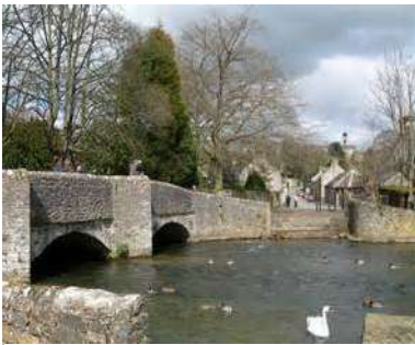
Bridge at Ashford in the Water
